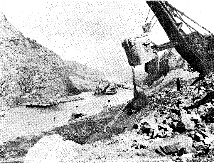
A steam shovel is hard at work on the west bank of Gaillard Cut in June, 1914. Cucaracha slide can be seen in the distance.
