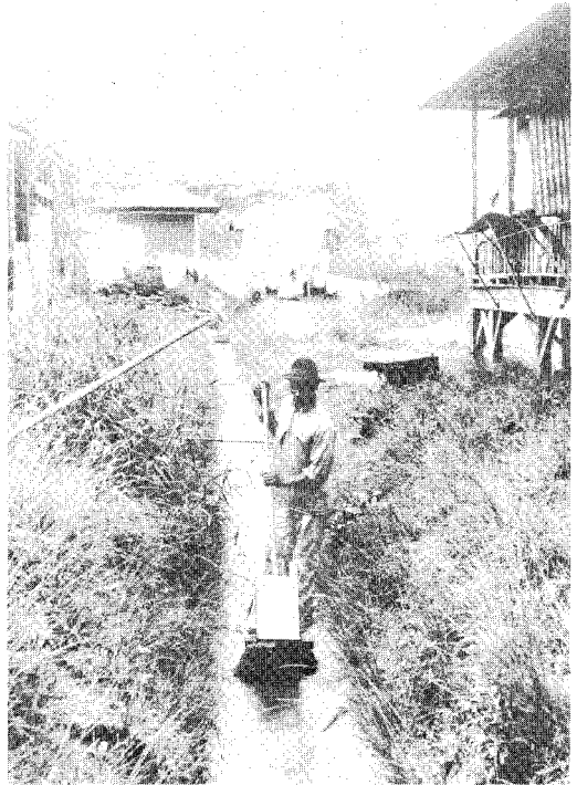
A notable achievement during Canal construction was the eradication of malaria, which is transmitted by the Anopheles mosquito. Here a larvicide is applied to a ditch as part of a mosquito control technique.
